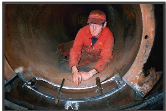
D-Patch Repairs
