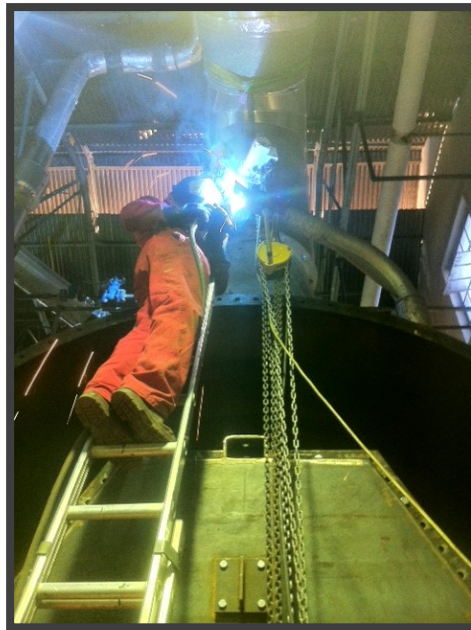
Structural Boiler Repairs
