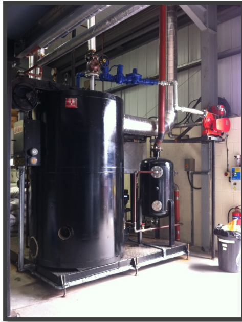
Skid-mounted Boilerplant
